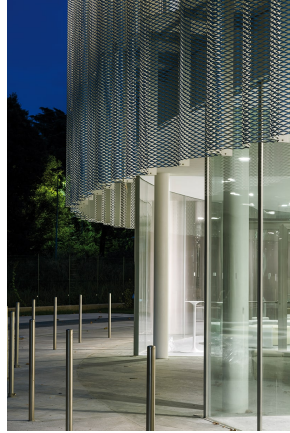
Figure 1. An example Permeable Double Skin Façade
